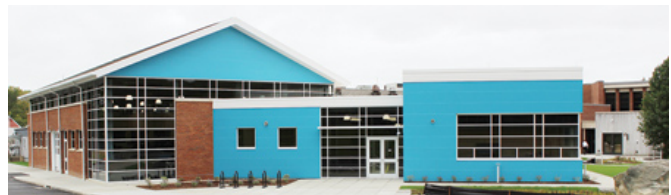
Designed by architects Silver/Petrucelli & Associates, QVCC Advanced Manufacturing Technology Center building is LEED Silver Certified and includes a machine shop lab, classroom, conference room, mechatronics and metrology labs, mechanical and IT rooms, and a tool crib.
